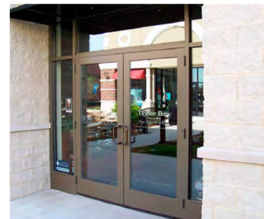
7. ALUMINUM STROEFONT SYSTEM BRONZE/DARK BRONZE
