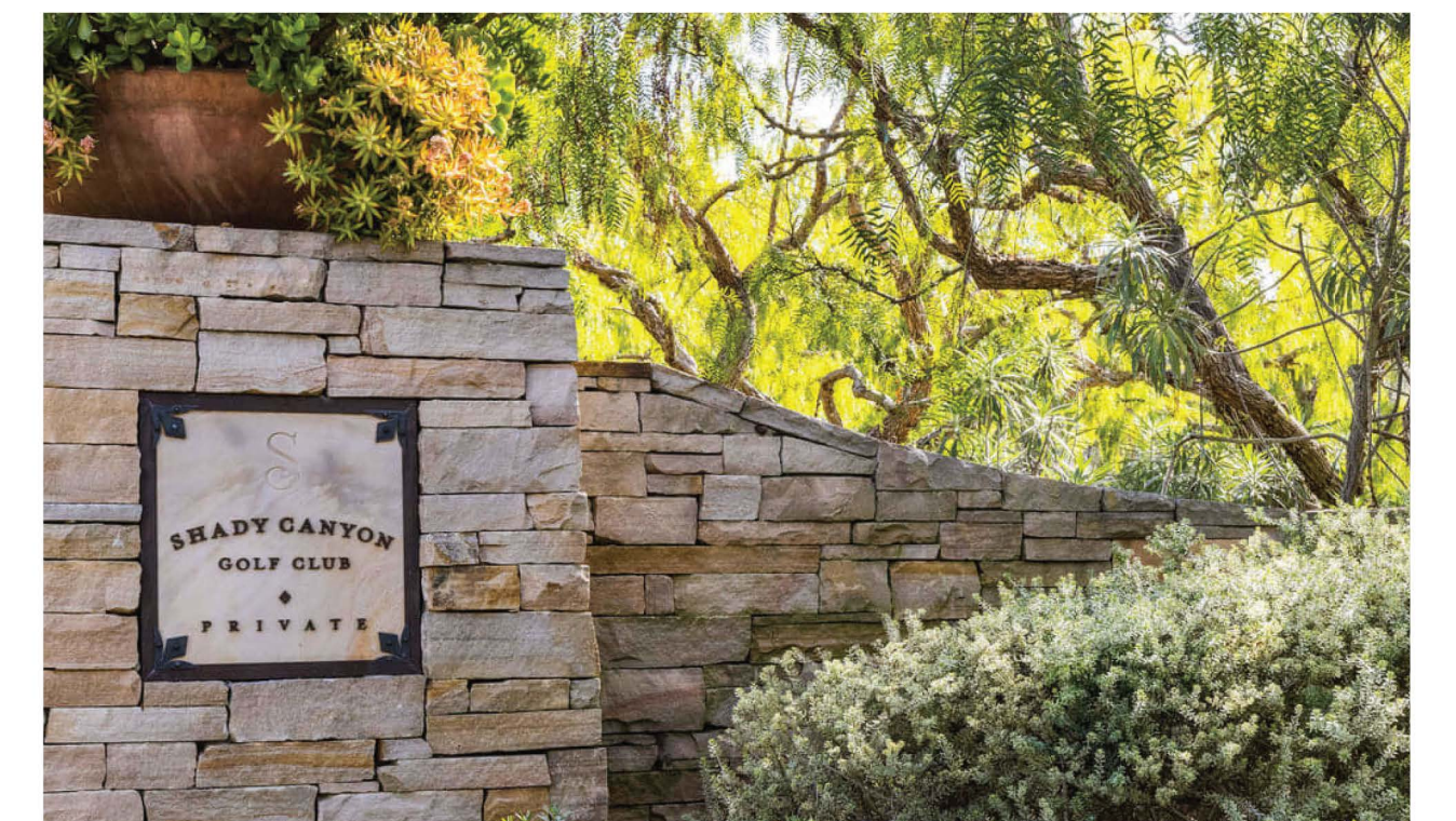
STACKED STONE WALLS & PILASTERS
