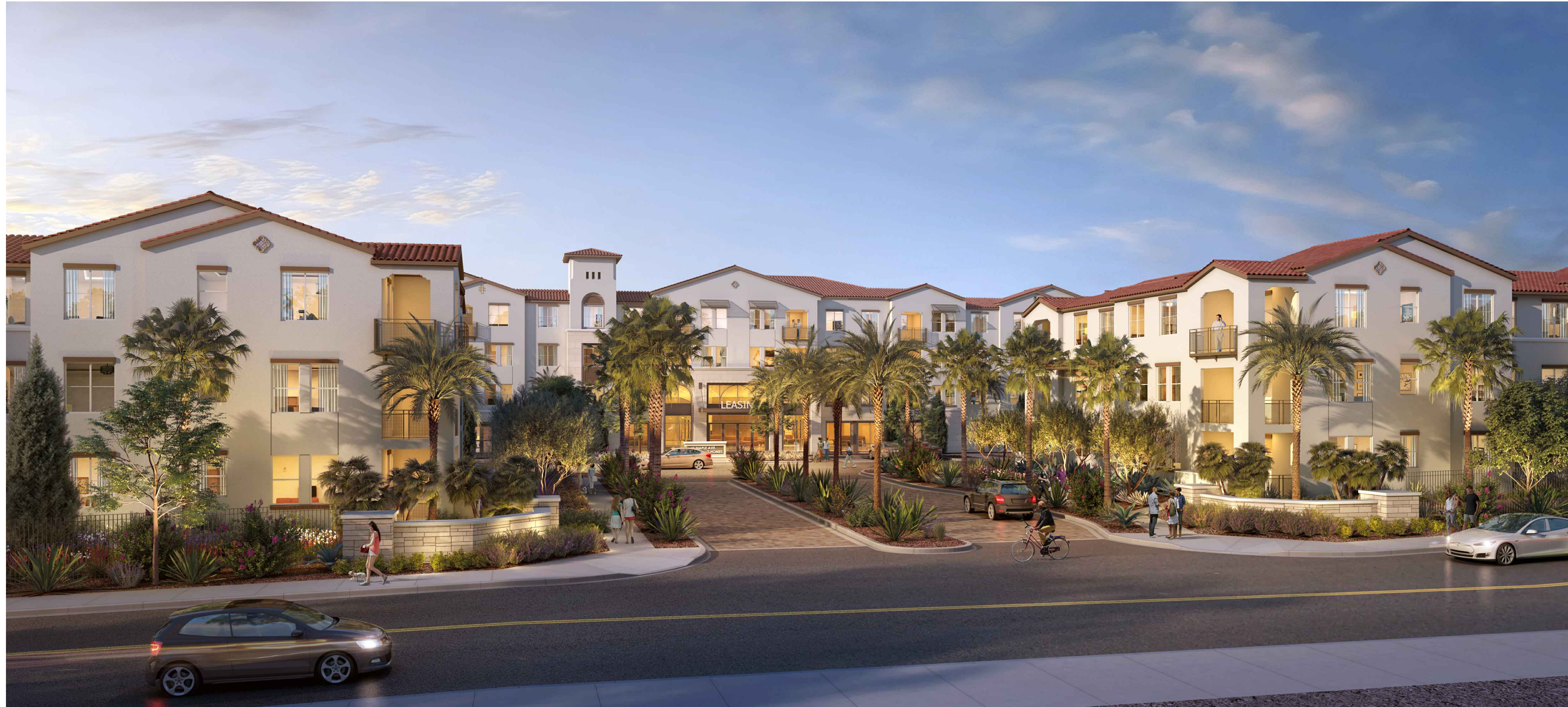
VIEW ON MAPLE LOOKING WEST 1
