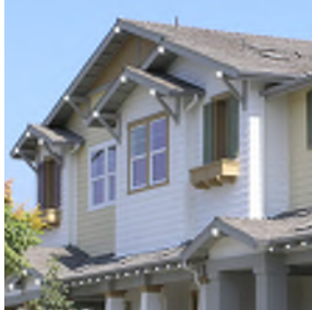
Exposed rafter tails at selected locations
