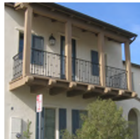
Wood corbels and balcony railing
