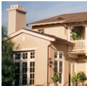
Shallow roof pitch, gable roof
