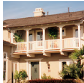
Exposed rafter tails at selected locations
