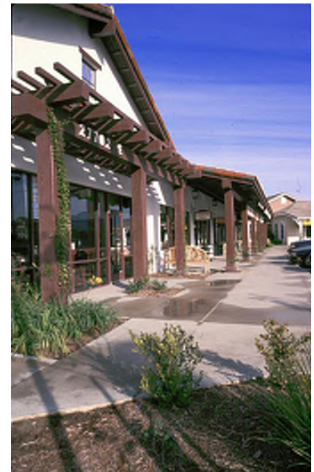
Distinctive architectural detailing
