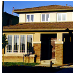
Heavy square columns
