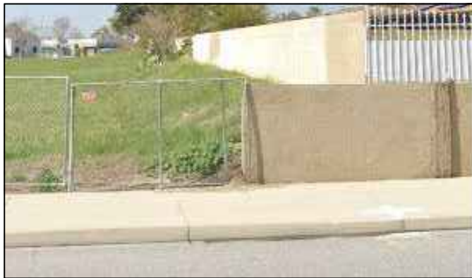
Citrus Ave. - north end Adjacent masonry wall
