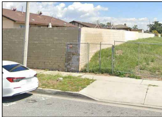
Tokay Ave. - north end Adjacent masonry wall
