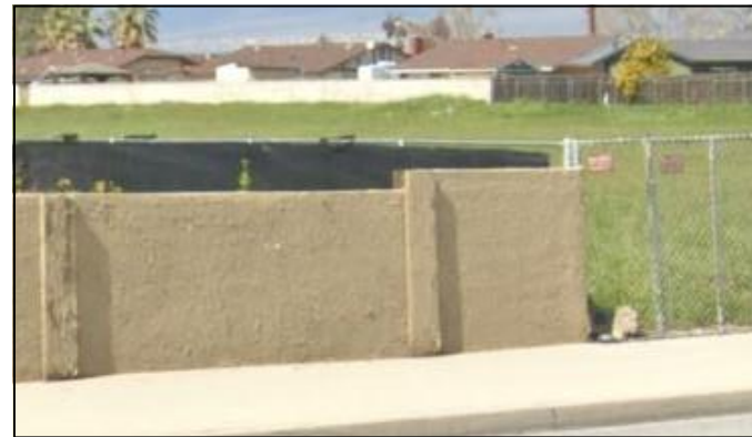
Citrus Ave. - south end Adjacent masonry wall
