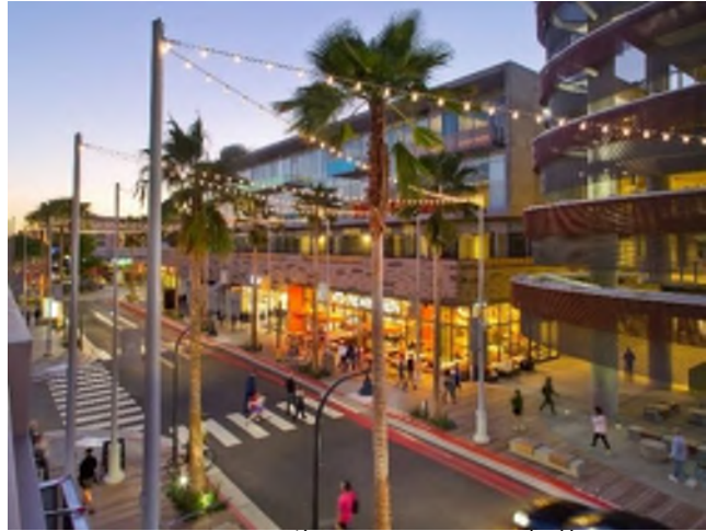
ground floor and residential above
