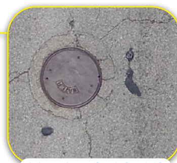
ASPHALT CRACKING
