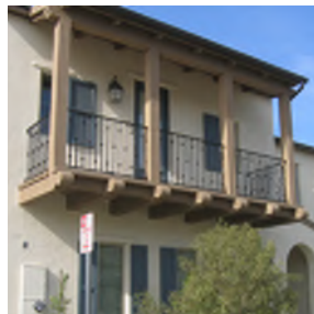
Wood corbels and balcony railing
