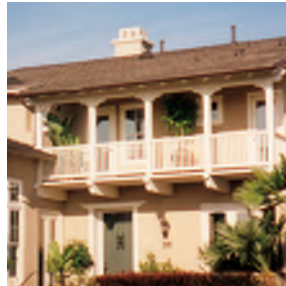
Exposed rafter tails at selected locations
