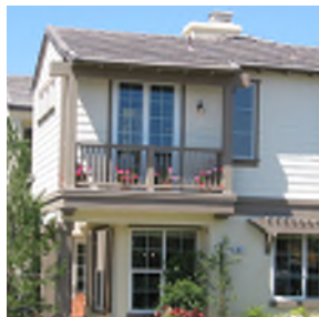
Accent siding at second floor
