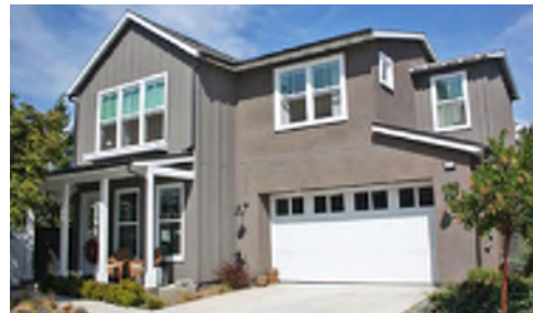
Covered entry with single story porch
