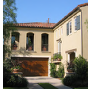
Asymmetrical building massing
