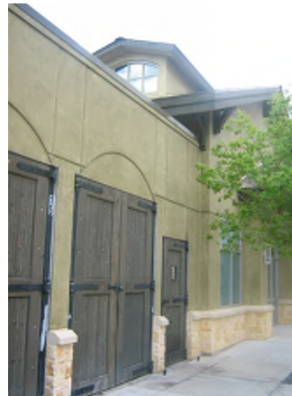
Screening of trash receptacles
