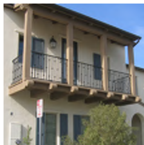
Wood corbels and balcony railing
