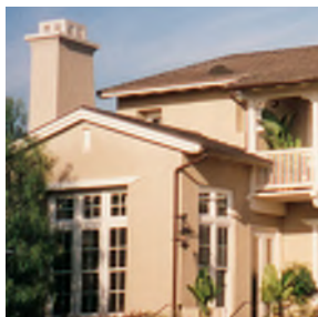
Shallow roof pitch, gable roof
