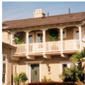
Exposed rafter tails at selected locations
