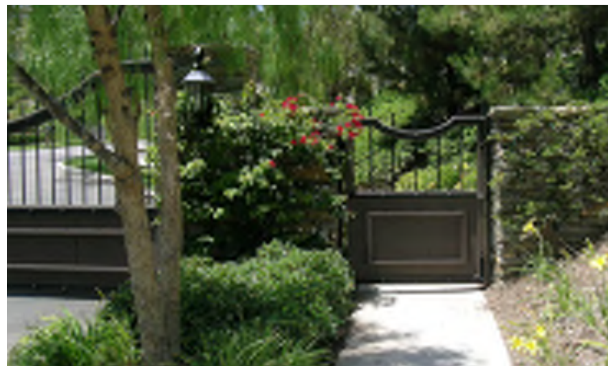
Example of pedestrian accessibility at gated entry
