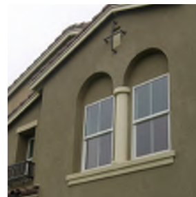
Arched windows & window treatments
