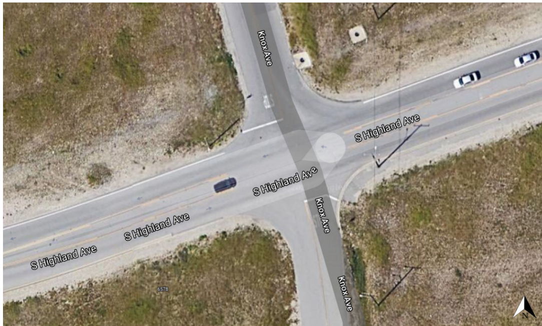
Figure 6.34: An Aerial View of the intersection of S Highland Ave & Knox Ave
