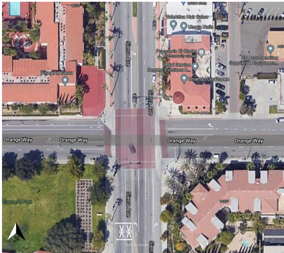
Figure 6.19: An Aerial View of the intersection of Sierra Avenue and Orange Way
