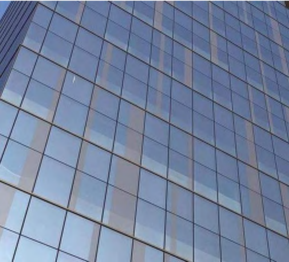
Exterior Glazing Viricon 1" Insulating Glass Unit VRE-4725
